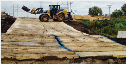
Bolted timber mat
