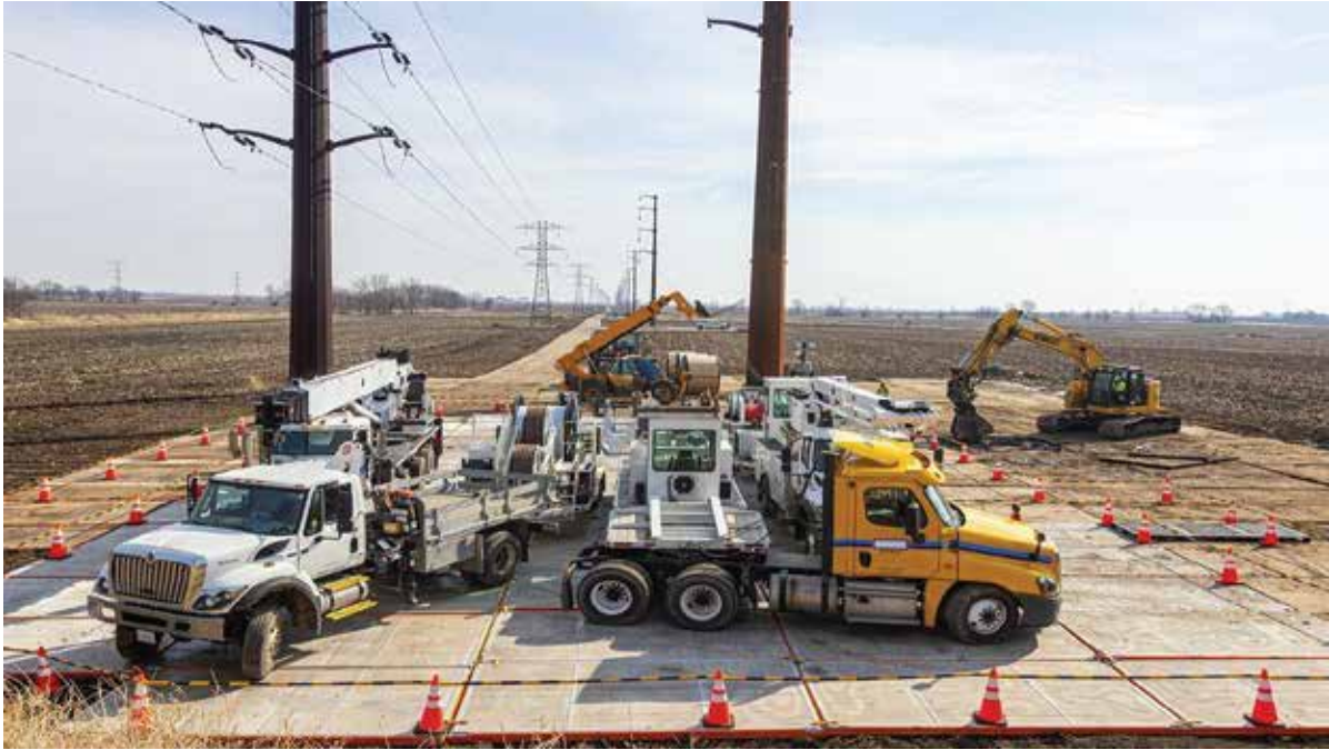
Example of an installed TerraLam EPZ Grounding Mat system that is in use
