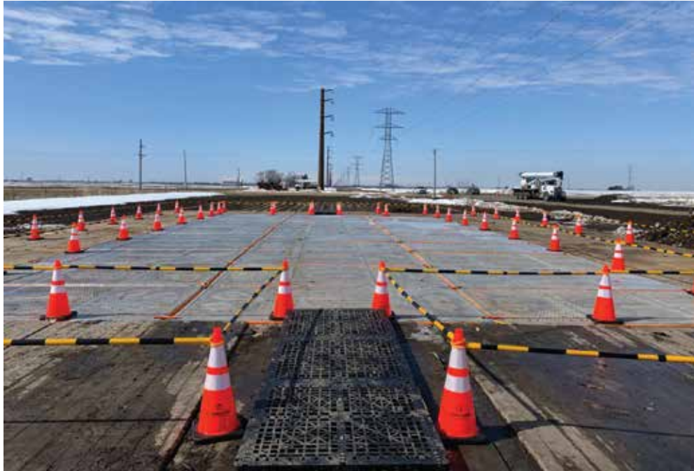
Example of an installed TerraLam EPZ Grounding Mat system
