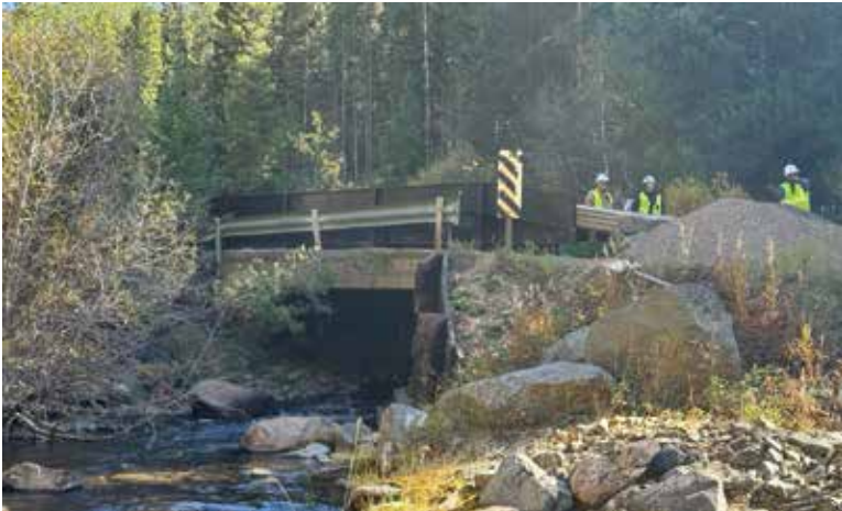
TerraCross bridge being used over an existing low, capacity bridge.
