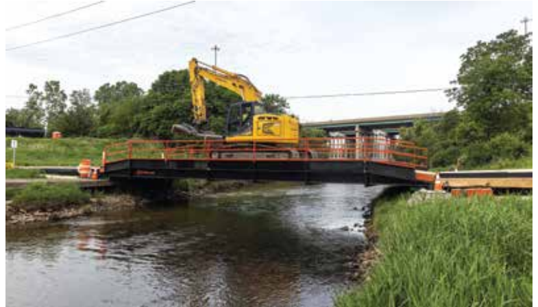
TerraCross bridge being used to cross over river without an existing bridge or crossing available.
